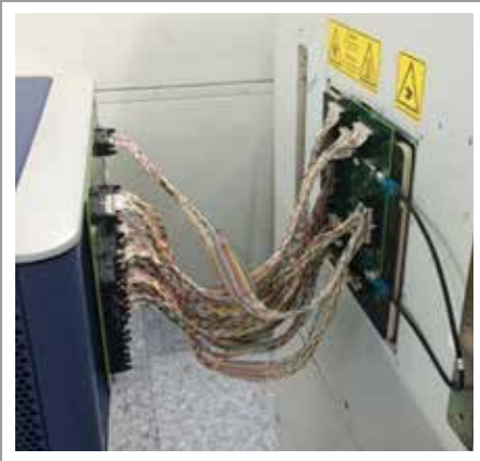
Old setup: Cable docking
